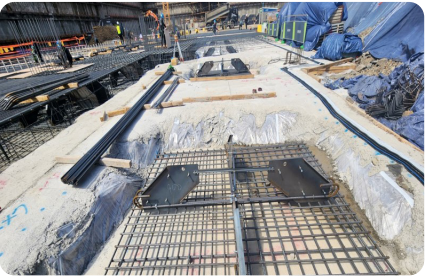
H Apartment in Daemyeong-dong, Daegu (Isolated Foundation, 1-leg Type)
